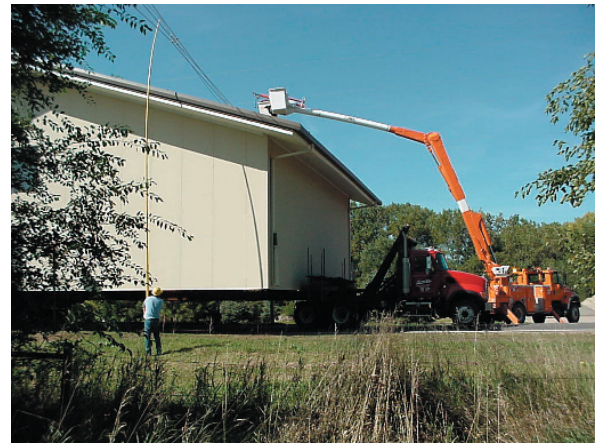
ERPPD personnel assisting with a building move near Battle Creek.
